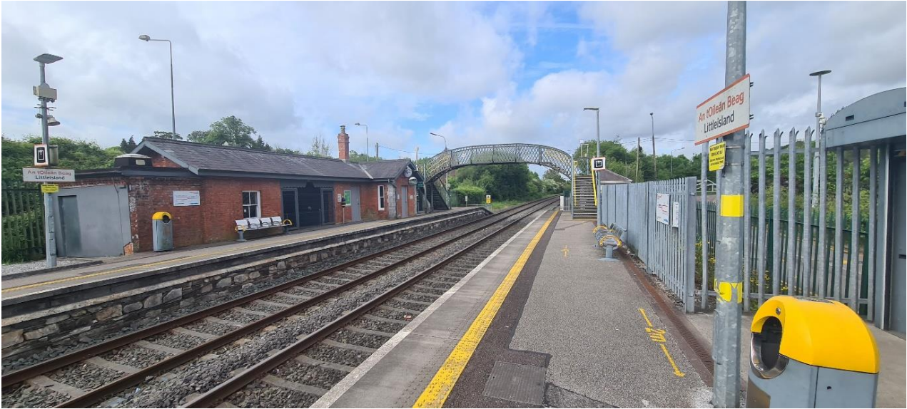
Photograph 8.8: View looking west from Little Island train station with Victorian station building and cast-iron footbridge and Proposed Development site beyond
