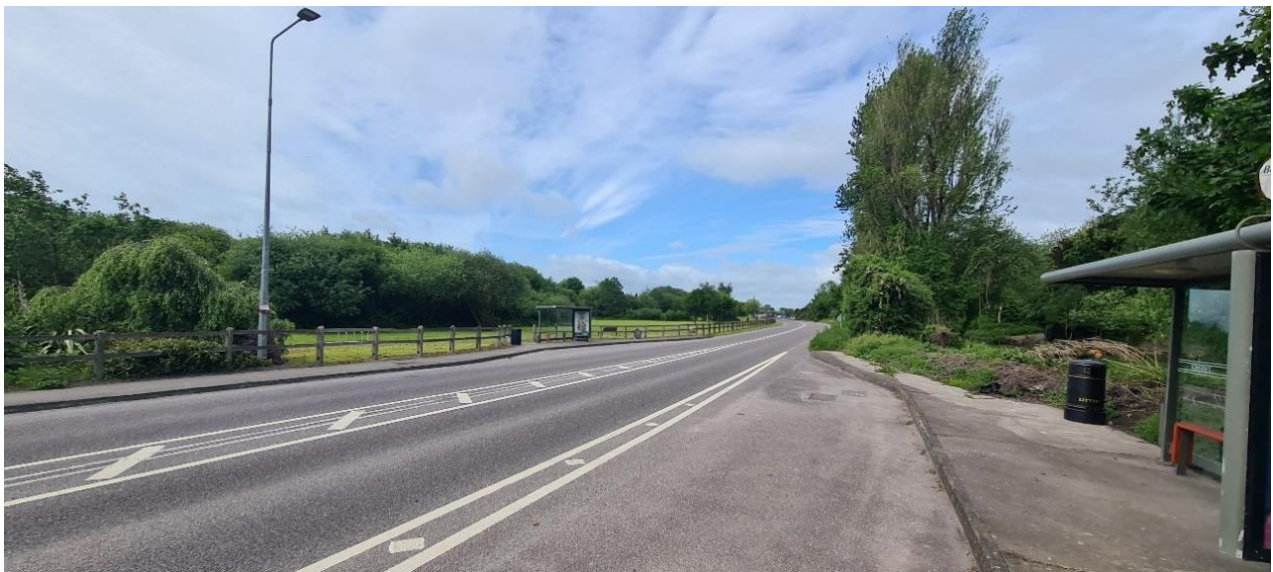
Photograph 8.4: View looking west on L3004 opposite junction with Little Island train station access road. Bus stops to both sides of road, mature trees and open space bounded by concrete post and rail fence
